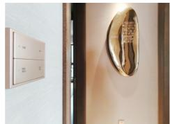
The panel is from the brand Inspid, which also uses KNX protocol. With only one panel, households can control the air condition, heater and lighting, which is easy and convenient for use. In this way, households would not be confused with countless buttons normally needed, and it also matched with the stylish interior design.
