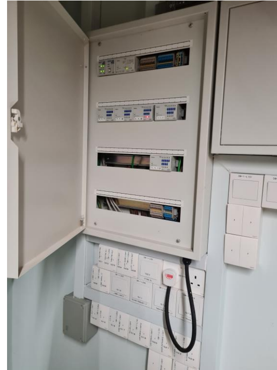
KNX Panel @ Ground Floor
