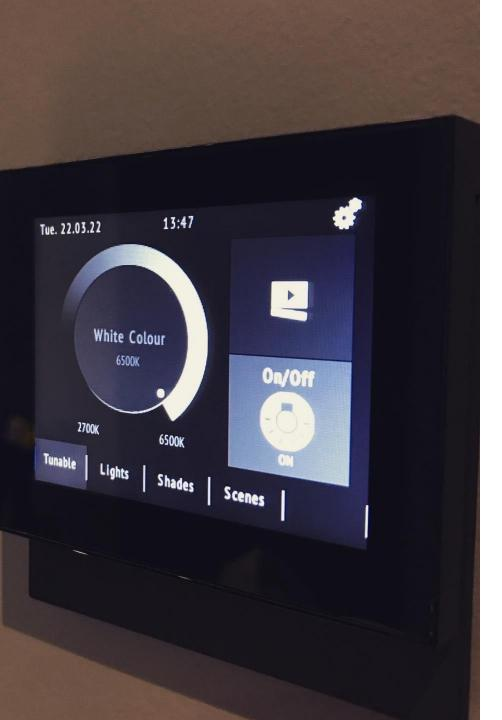
The user can choose between 2700K and 6500K color temperature for the DALI lights of the apartment. Besides the manual control, the color temperature is adjusted automatically according to the time of day following 8 specific presets. So, every time the user turns the lights ON, the lights will automatically adjust their color temperature based on what time it is.
