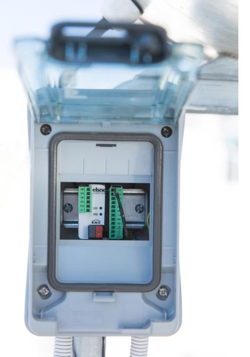
The domestic hot water temperature is monitored and recorded by ELSNER's evaluation unit via a T130 sensor. Additionally, we have created a threshold switch function of the measured temperate in order to trigger the recirculation of the hot water using minimum and maximum values. That way the user will always have hot water available instantly.
