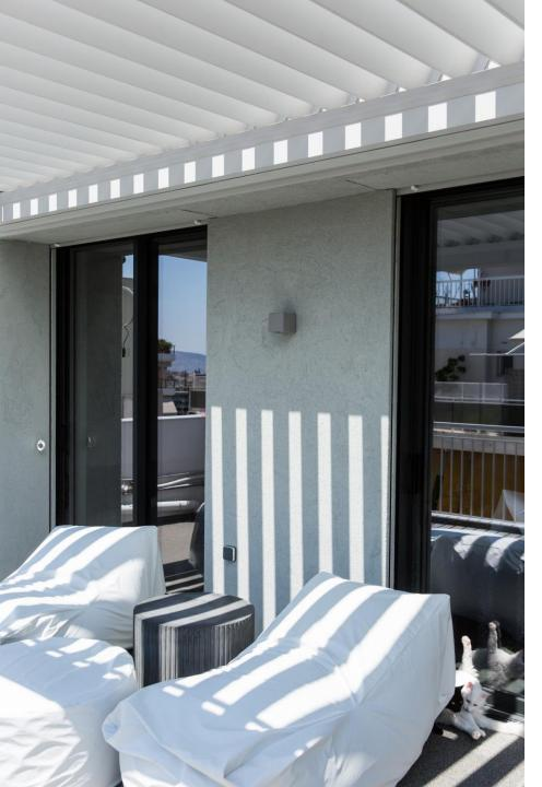
With the help of the weather station, the louvers are being controlled according to the azimuth and elevation values of the sun.
