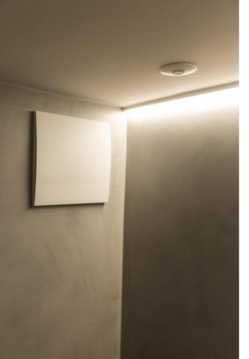
Every bathroom is equipped with LUNOS silvento ventilation systems. A presence detector automatically turns on the DALI lighting and starts the ventilation. The ventilation function has been programmed with retriggering events and a timer of 5 minutes delay after the presence is no longer detected.
